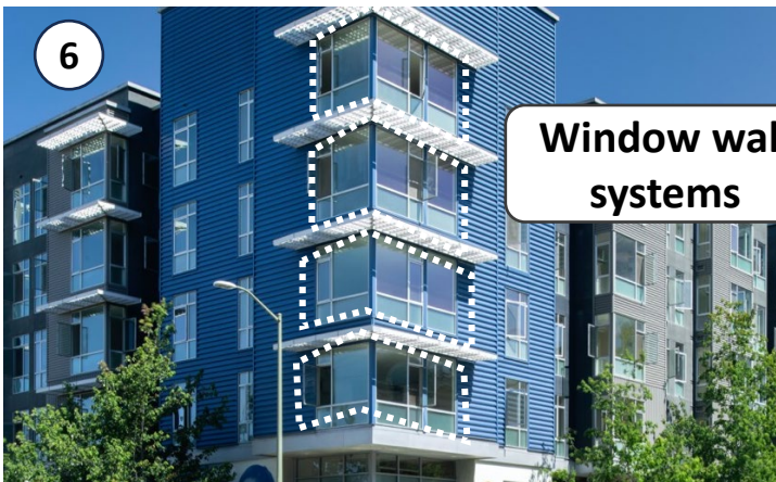
6. Window wall systems (full glass and metal panels) at the corners.
