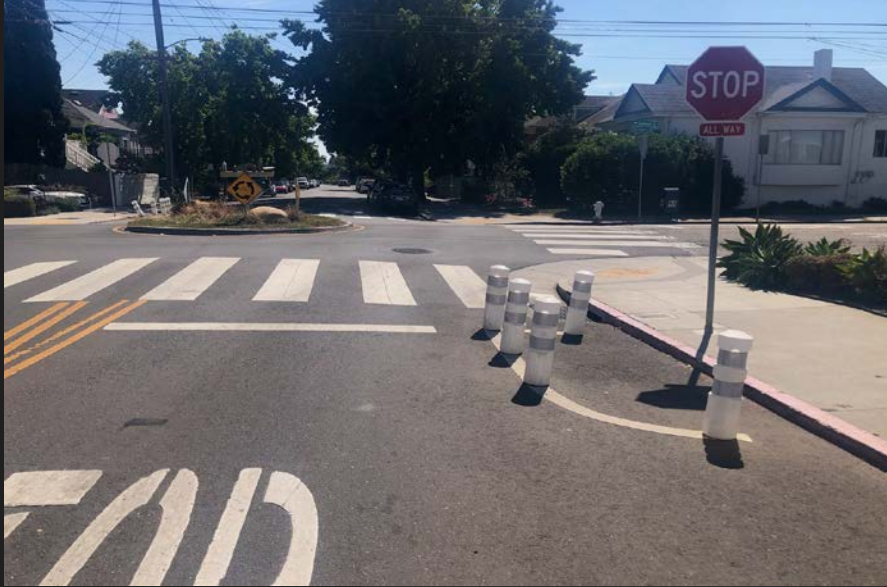
Shafter Ave, Oakland Example of bulbout using wide flexposts
