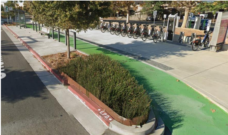
Floating with raised (sidewalk-level) bikeway
