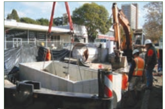
Installation of a trash separator
