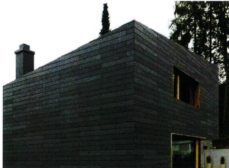
HORIZONTAL FIBER-CONCRETE BOARD RAINSCREEN SYSTEM
