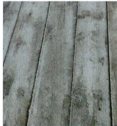
CLEAR-SEALED BOARD-FORM CONCRETE COLUMNS
