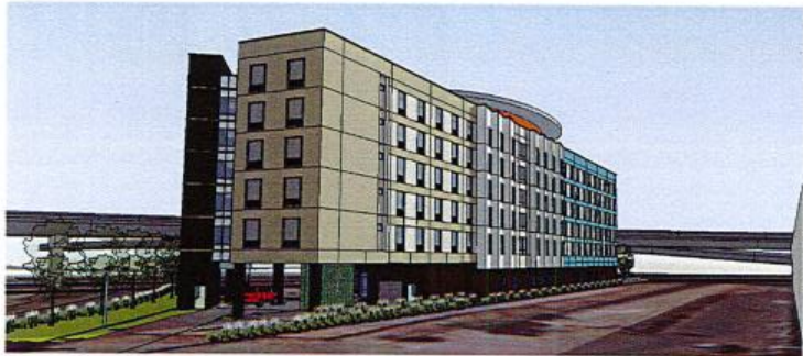
North East View - Side
