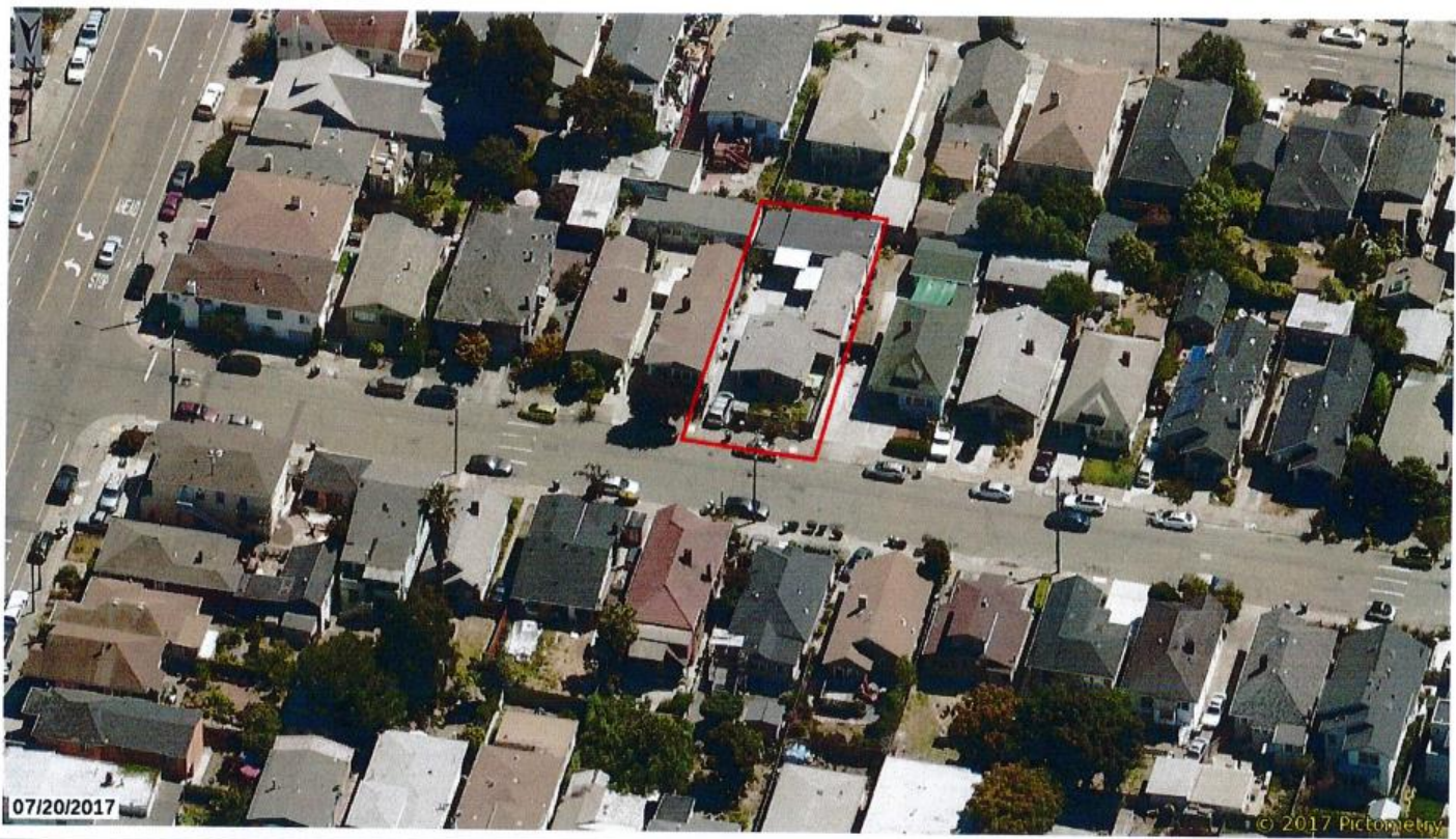
Aerial image showing the north elevation. The subject site is indicated in a red outline.
