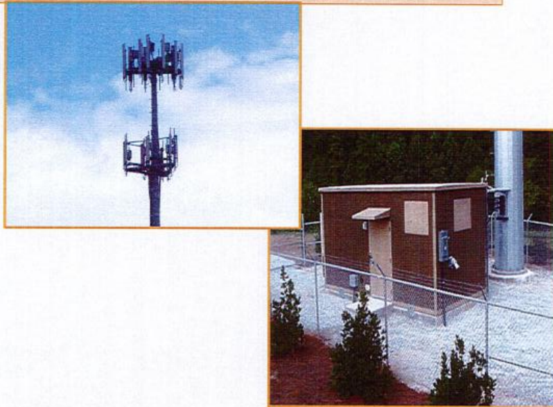
Typical Macro facility – industry standard sized collocateable facility with full compliment of radios
