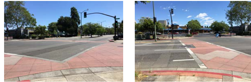
Exhibit I-2B: Faded Crosswalk; Median With No Refuge Island
