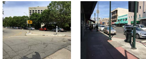
Exhibit C-4A: Pedestrian Refuge Island With No Crosswalk; Pole With No Pedestrian Activation Button
