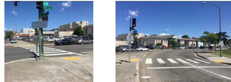
Exhibit I-3B: Pole with No Pedestrian Countdown Timer; Channelized Right Turn Lanes
