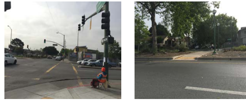
Exhibit C-5A: Crosswalk Adjacent to School With No High Visibility Markings; Mid-Block Curb Ramp With No Crosswalk
