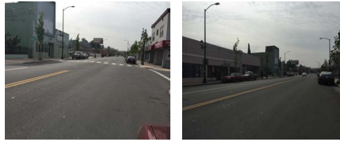
Exhibit C-3A: Four-lane Road With No Crossing; Mid-Block Crosswalk With No Advanced Yield Markings
