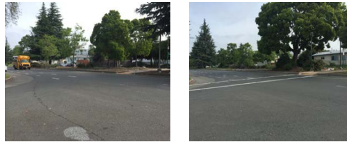
Exhibit C-10A: Mid-Block Curb Ramp With No Crosswalk; Crosswalk With No Signage
