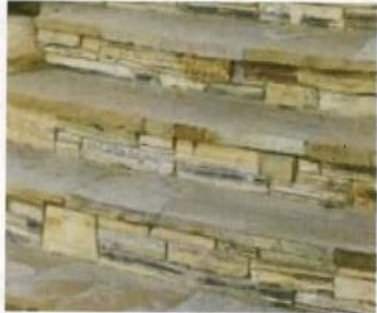
① STONE CLAD STAIR
