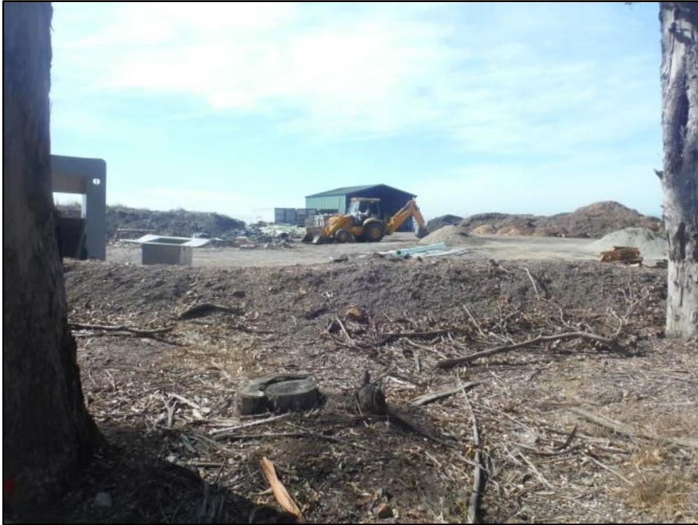
Photo 1: View SW, Construction yard at NW corner of New Plot 82.
