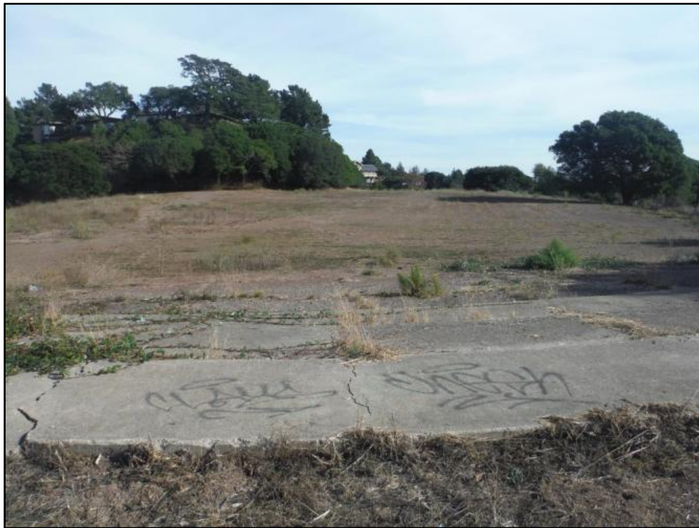
Photo 8: View SE, Showing stepped semi-circular concrete structure and asphalt slab.
