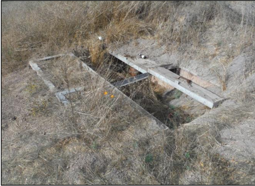
Photo 7: View N, showing board-formed vault with water main.
