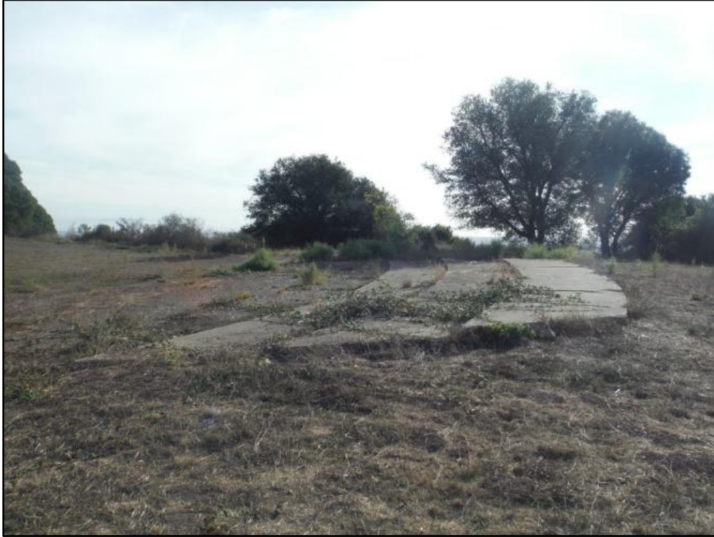
Photo 9: View S, showing concrete stepped, semi-circular structure and asphalt slab.
