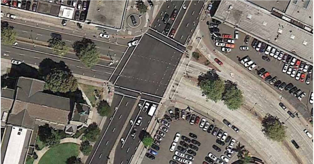
Aerial View - Existing Configuration
