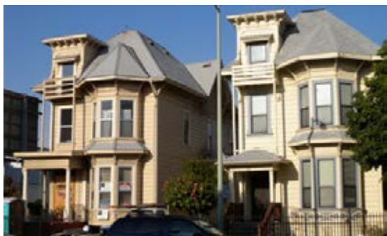
The Stick-Queen Anne Style Real Estate Union Houses feature hip roofs, polygonal bay windows, covered entrances, ornamental wood paneling, and decorative roof cornice support brackets.
