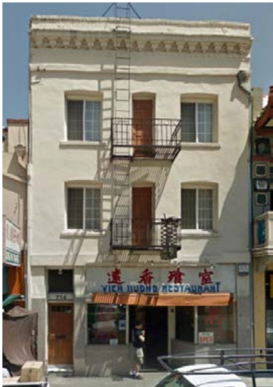
Well-articulated facades create a clear distinction between the ground floor and upper stories.
