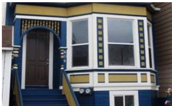
Recessed entrances with overhanging arches and spindlework and polygonal bay windows characterize many of the area's late 19th century residences.
