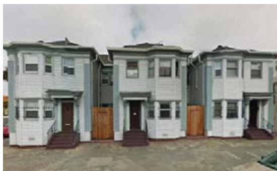
Though modified over time, this attached triplet of Colonial Revival duplexes is significant for its ingenious adjoined structure.
