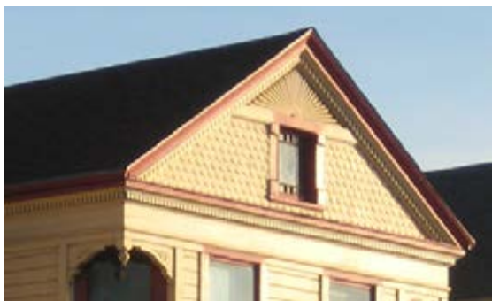
Attic windows, sunburst apices, fish-scaled shingles, dentils, and ornamental corner support brackets are character defining features of Queen Anne style residences in the District.
