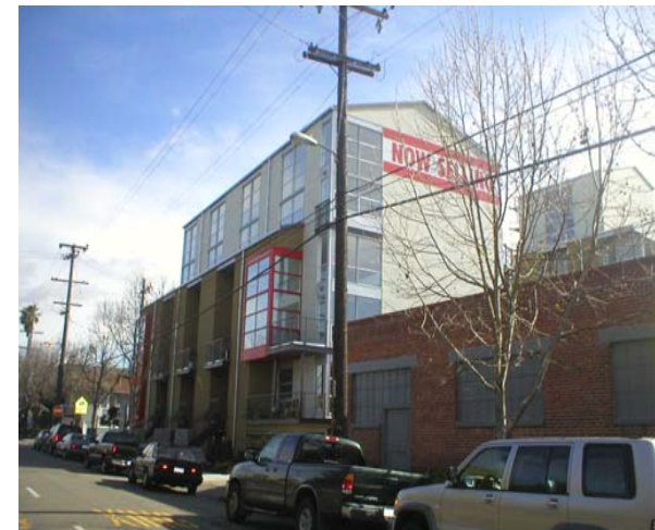
Guideline 4.1: Upper story stepbacks reduce the scale of a building appropriate for the width of a street and neighboring buildings.
