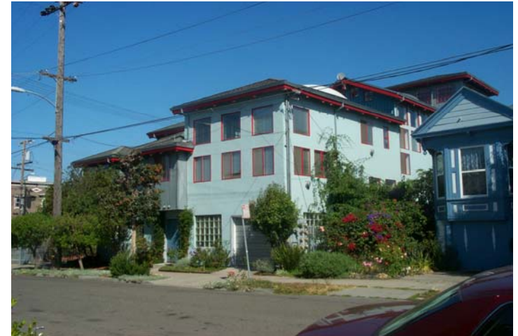
Guidelines 4.1 and 4.2: Variations in roofs height and upper story setbacks reduce the scale of this building and provide a transition to the neighboring smaller scale property.
