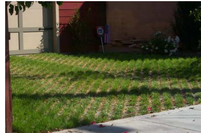
Guideline 8.3: Landscaped paving softens the appearance of outdoor parking areas and decreases off-site runoff.
