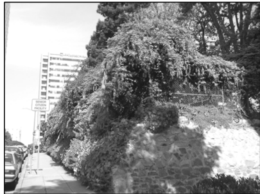
View of rock embankment
