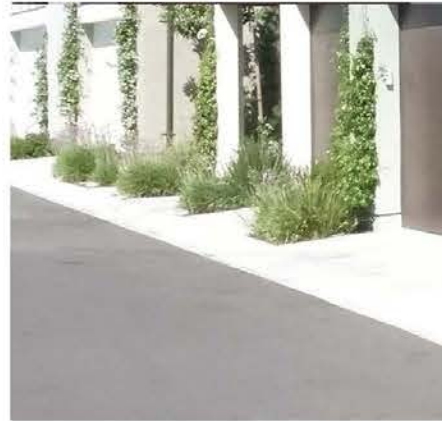
PRIVATE ACCESS DRIVE - ASPHALT DRIVEWAY WITH CONCRETE ROLLED CURB AT EDGE
