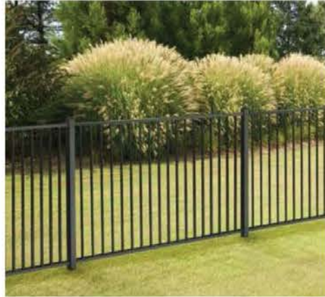
STEEL PICKET FENCE - 42" OR 6' TALL, SEE PLANS
