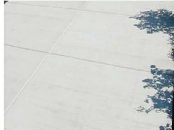
PEDESTRIAN PAVING - CONCRETE WITH BROOM FINISH
