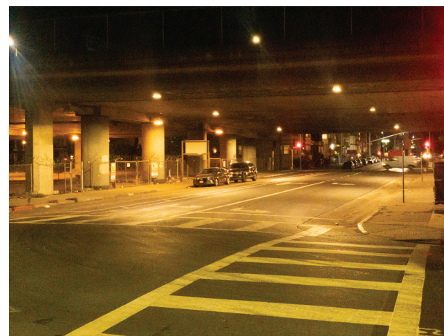
Typical existing nighttime conditions
