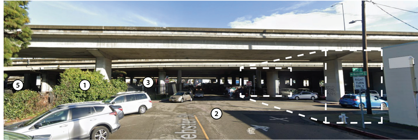
WEBSTER STREET UNDERPASS FACING NORTH
