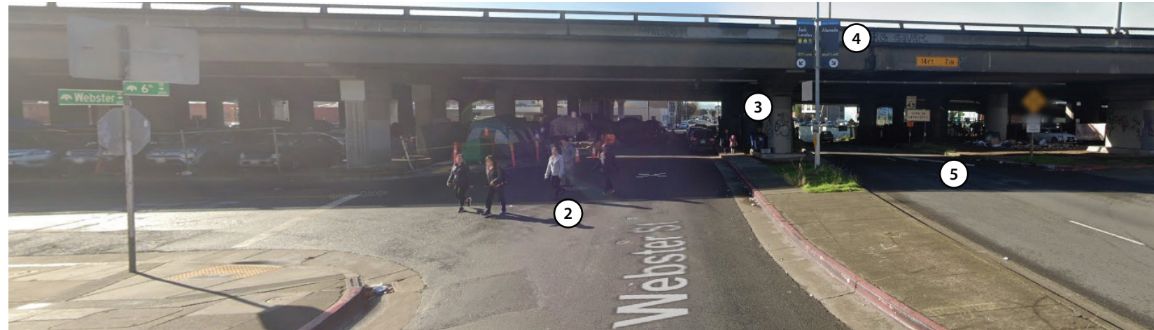
WEBSTER STREET UNDERPASS FACING SOUTH
