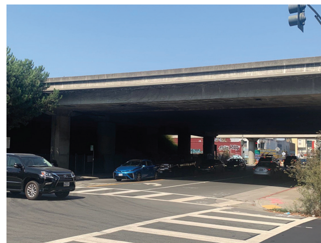
Example of dark embankment areas
