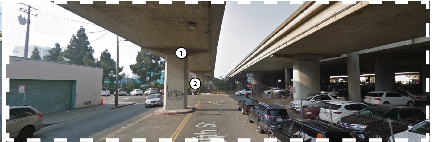
WEBSTER STREET UNDERPASS FACING WEST
