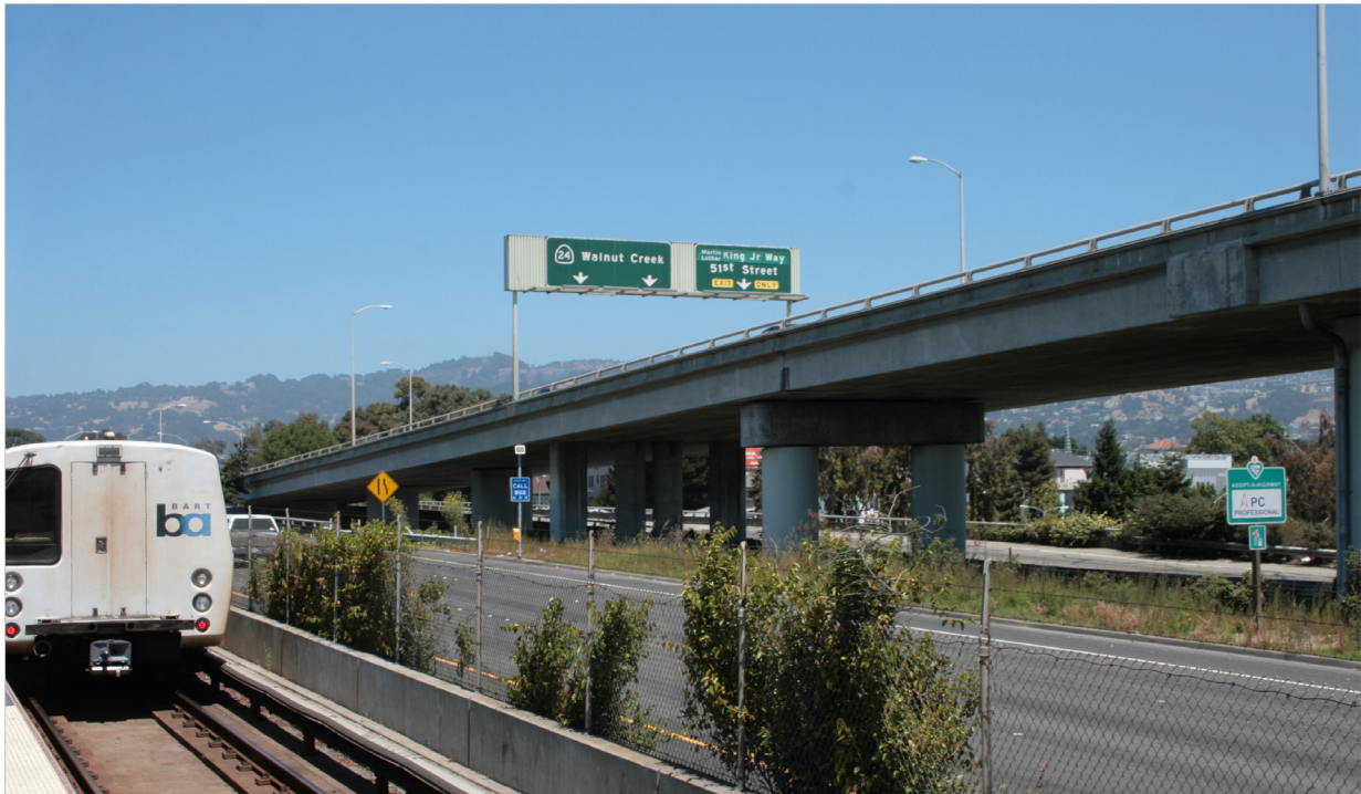
Existing view of project site from the MacArthur BART station platform (Viewpoint 5)
