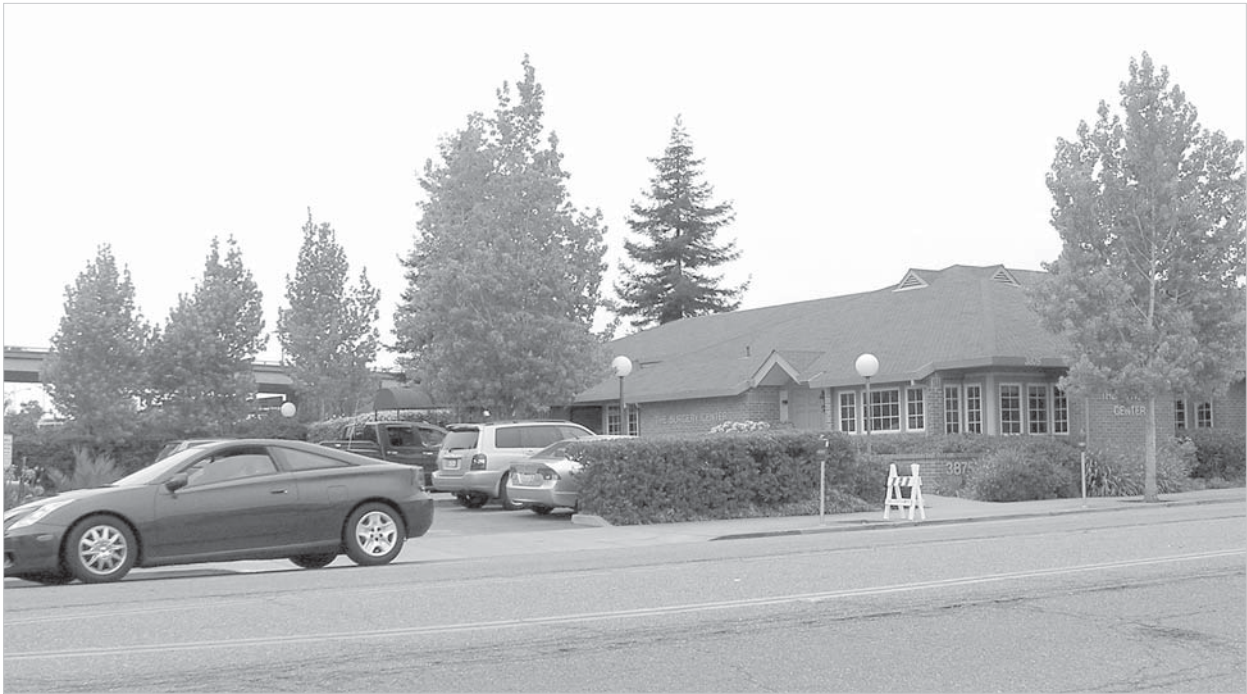
Photo 6: View looking west of the existing medical office on the project site
