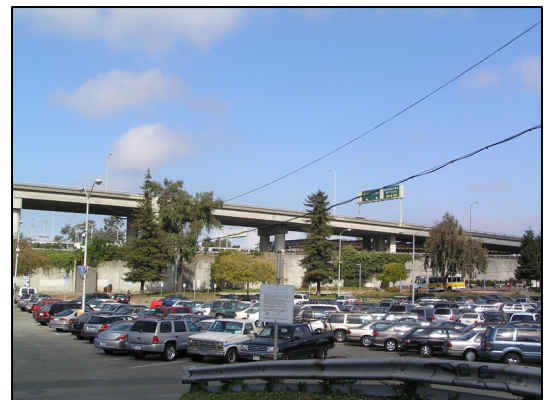
View of project site, looking west toward State Route 24.
