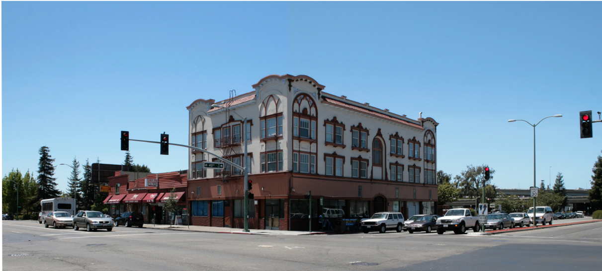
Existing view of project site from the intersection of Telegraph Avenue and 40th Street (Viewpoint 1)
