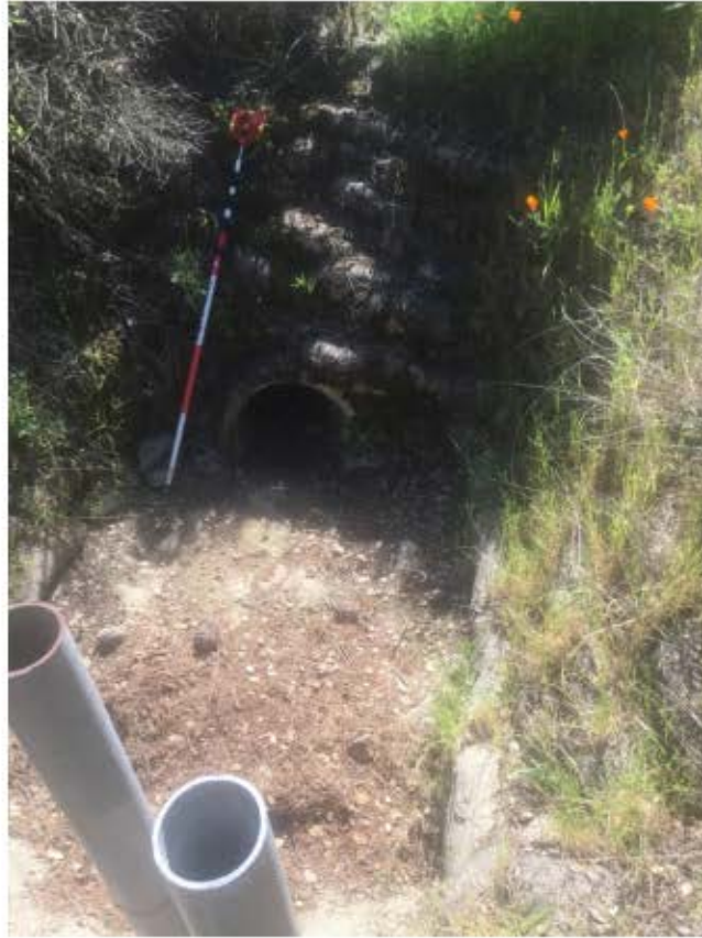
Photo 1 - Downstream sump and invert pipe (1.5 ft diameter, concrete) surrounded by headwall.
