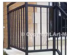
FENCE CONCEPT 3-1/2 FOOT HEIGHT WROUGHT IRON FENCE WITH GATES AND OPEN RAILS TO MATCH ENTRIES
