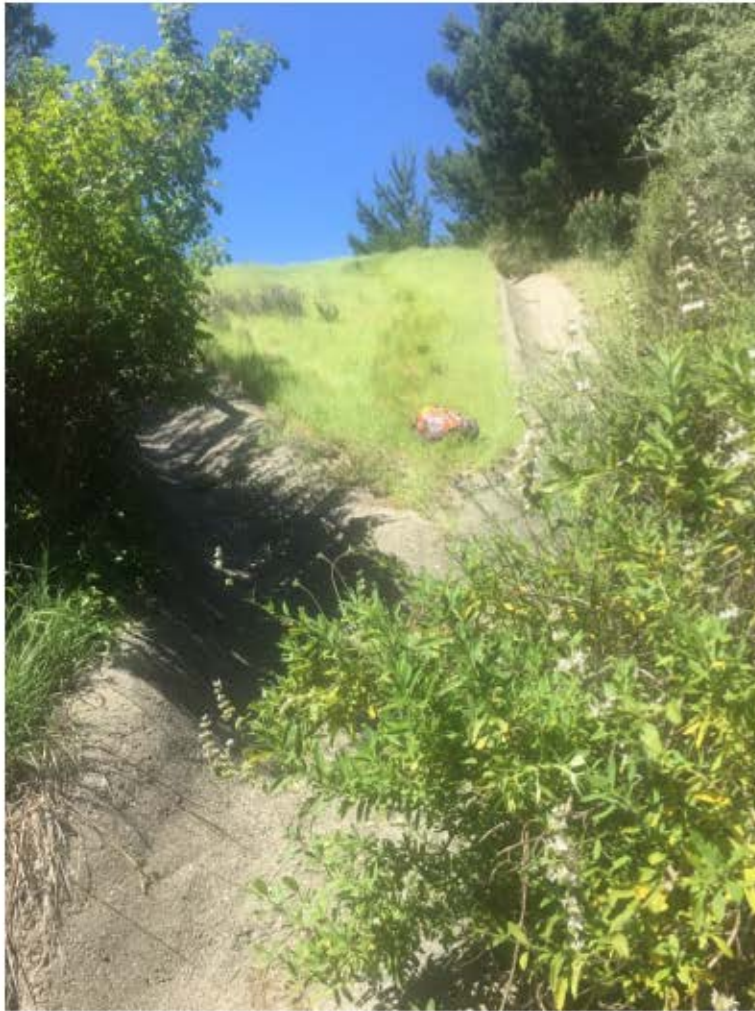
Photo 3 - Open concrete drainage canal.
