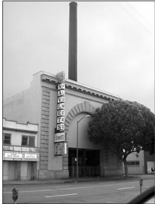
Great Western Power Company Building
