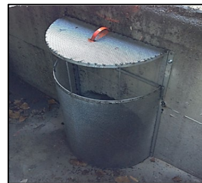
Full trash capture device covers pipe opening to block trash and let water through.
