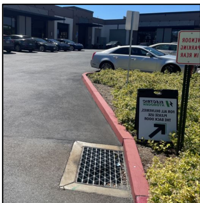
Photo shows a very clean property with a storm drain that connects to the City's system. This property is implementing effective BMPs.
