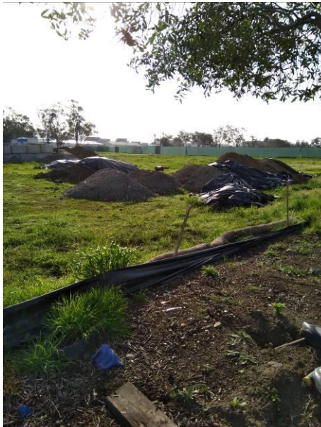
Photo #28 View of fill piles, located within the construction fence.
