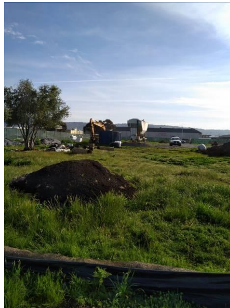
Photo #24 View of operations within the construction fence, facing east.
