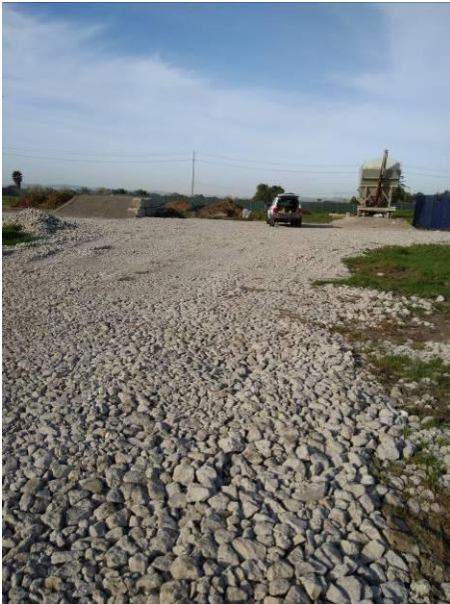
Photo #25 View of operations within the construction fence, facing west.
