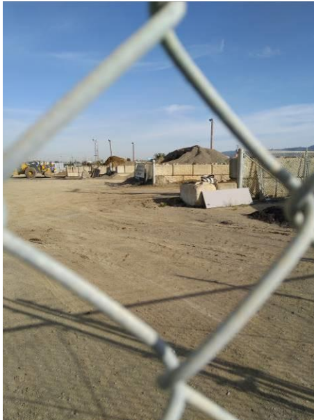
Photo #33 View of additional fill pits, located on the adjoining property to the north.
