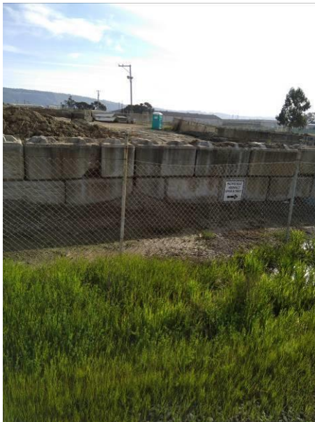
Photo #11 View of the northwest corner of the site, facing East (slurry pit area)..
