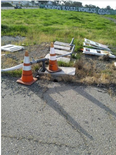
Photo #21 View of water connections, located on the northern portion of the site.
