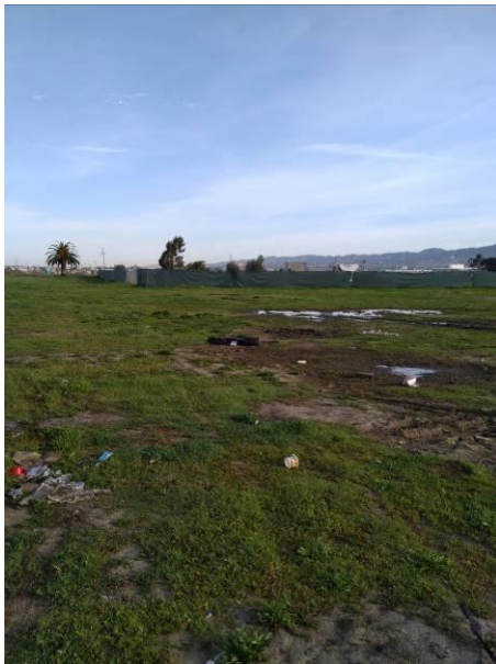
Photo #23 View of construction area fence boundary, located in the center of the site.
