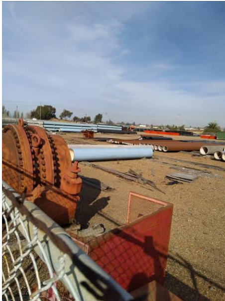
Photo #5 View of the northeast corner of the site and adjoining northern property, facing west.
