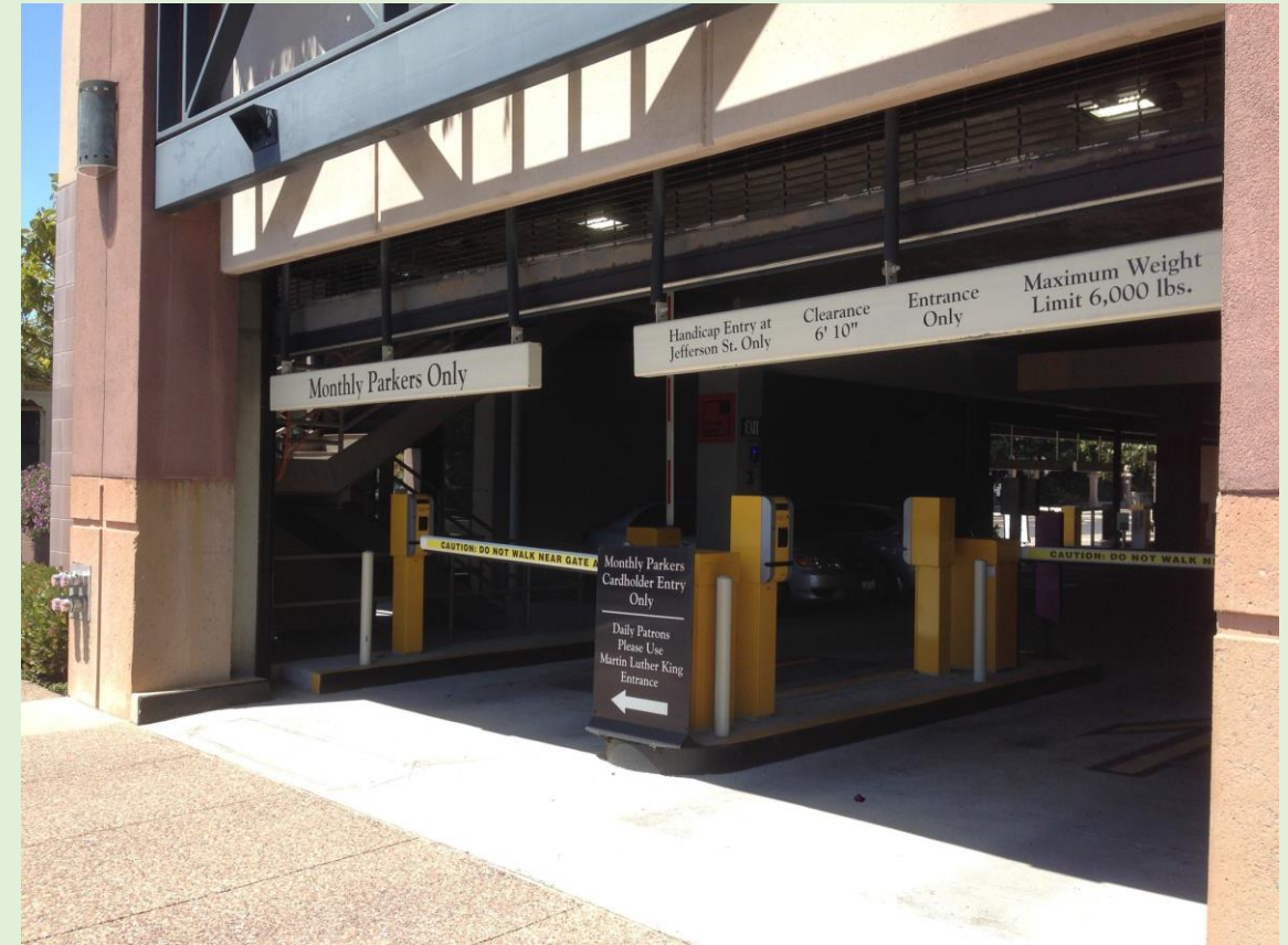
City Center West Garage Entrance
