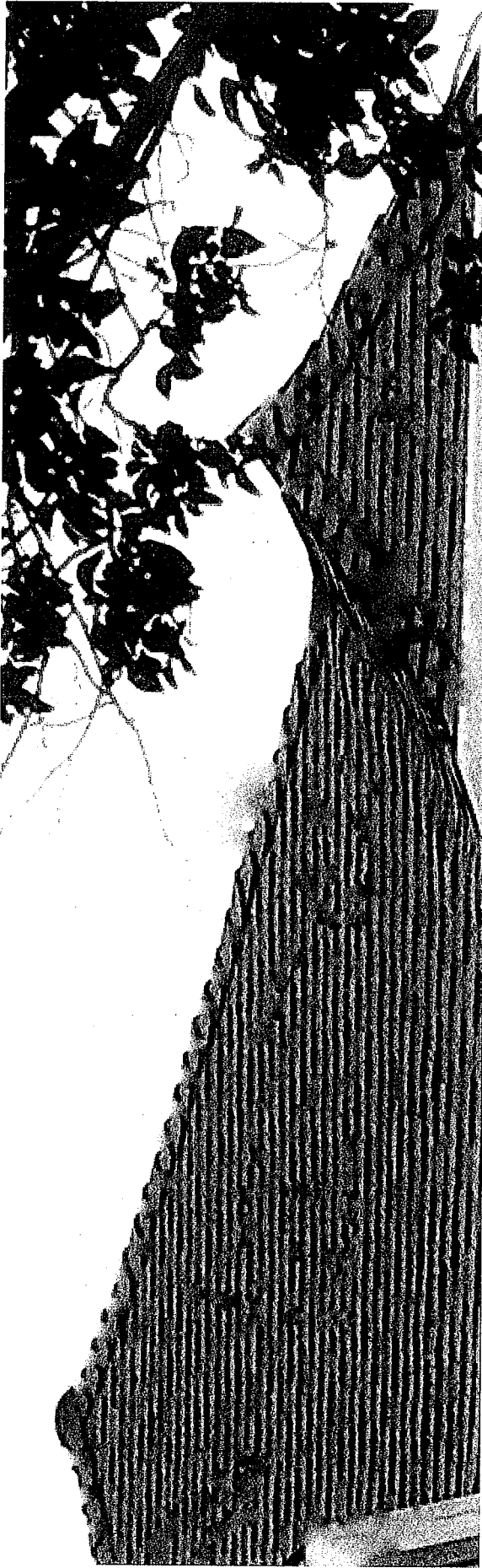
Image #7 Roof, gutters, down spouts and plywood replacement Years 2020-2022 of the work plan (sorry couldn't get a good picture of the roof)
