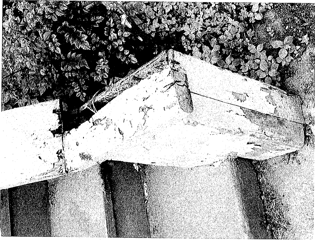
Image #2 Front stair wall to be rebuilt Years 2017-2019 of the work plan
