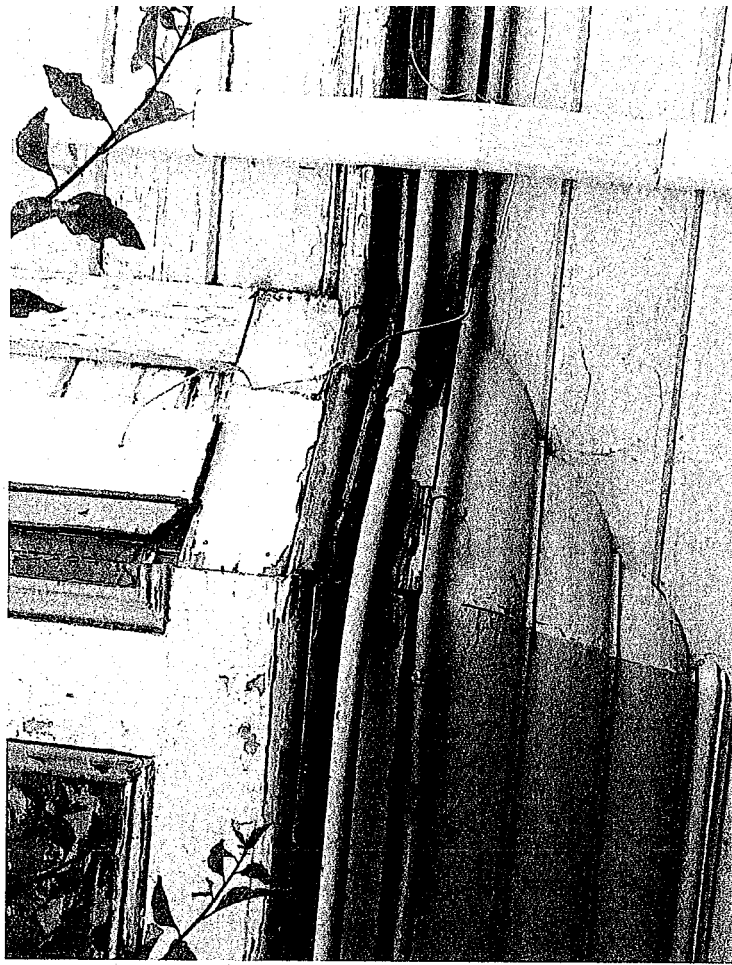
Image #4 Exterior dry rot, refastening and replacement of detailing (the whole house looks like this) Years 2017-2019 of the work plan
