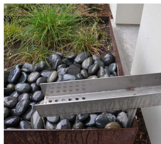
BIOREMEDIATION FLOW THROUGH PLANTER
