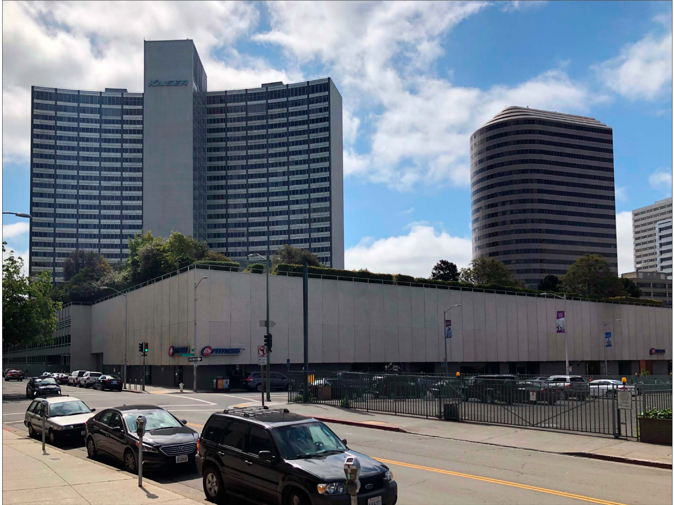
VIEW FROM 21ST / WEBSTER TO EAST
