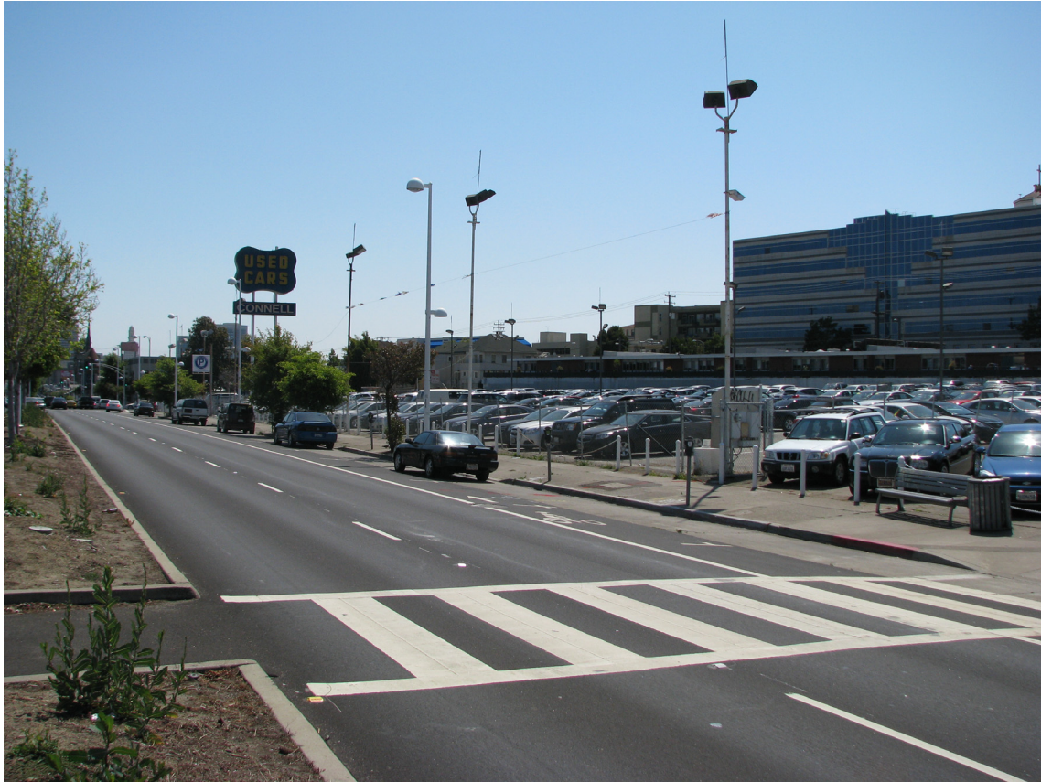
3 Looking southwest from Broadway at midblock
