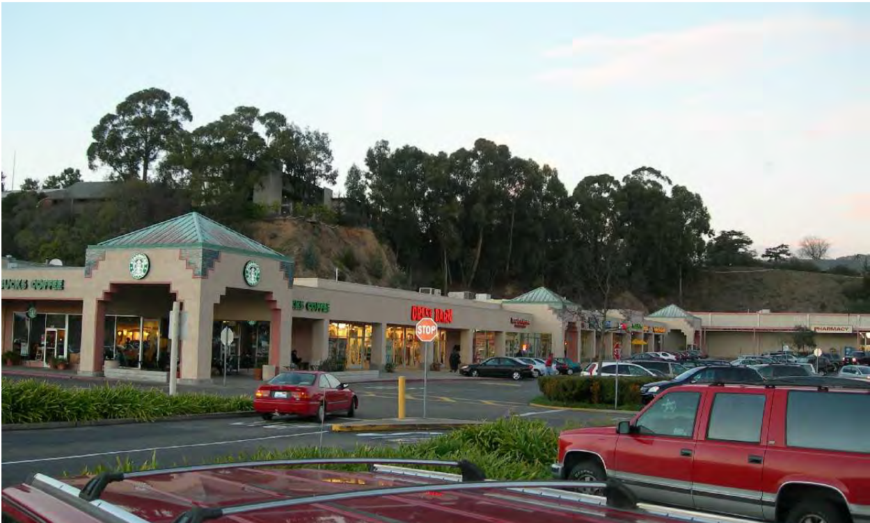
Photo 4: Central Building, Buildings 4
