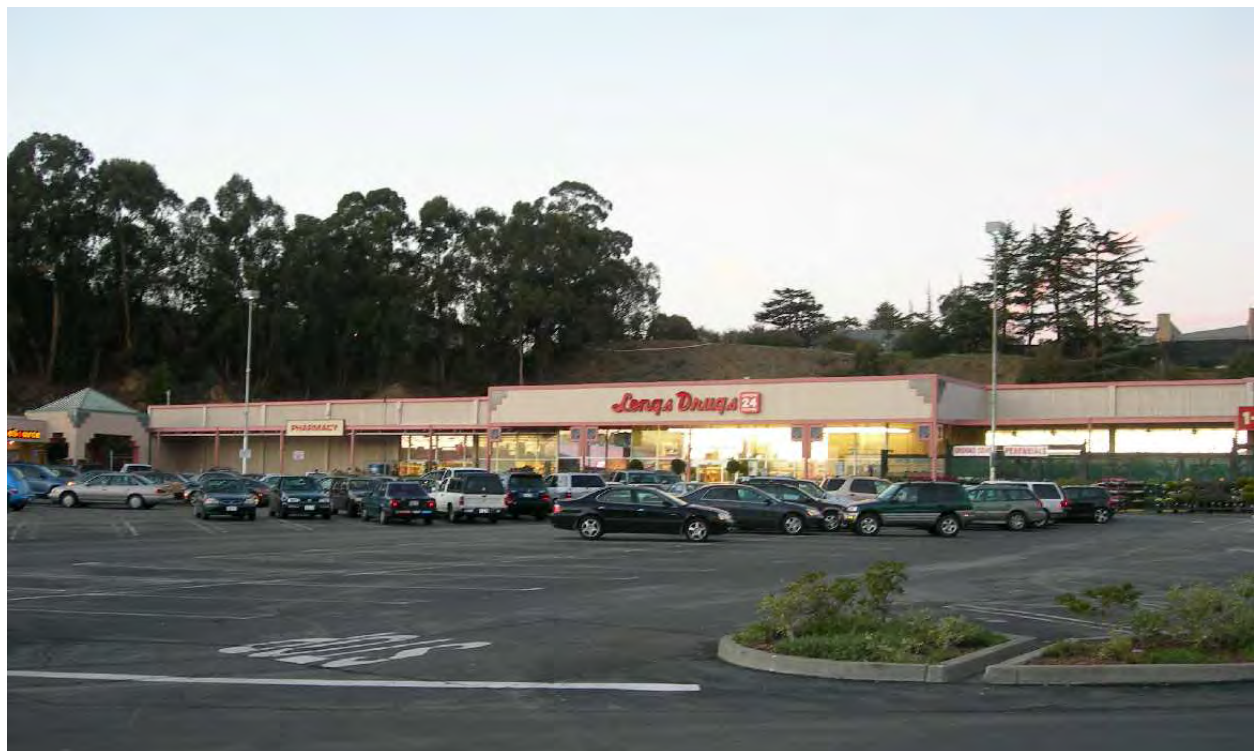
Photo 6: Existing CVS Pharmacy. Building 6 (was Long's Drug)
