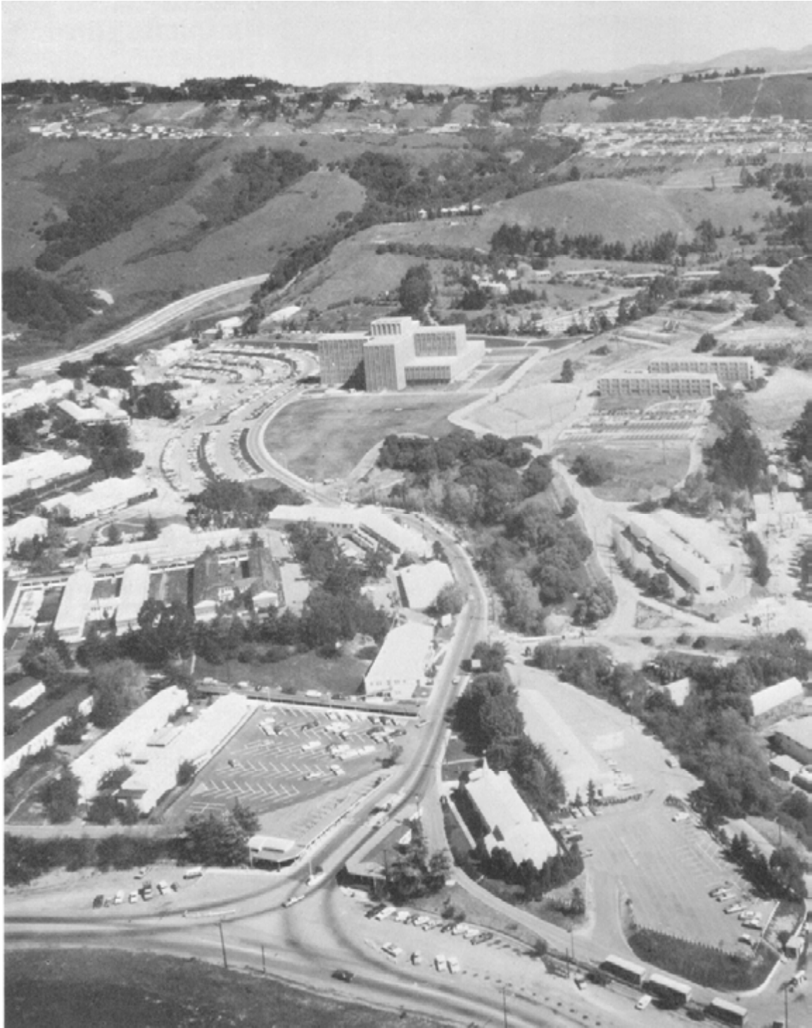
Figure 5. 1973 Photograph of U.S. Naval Hospital in Oakland. (Source: 1973 Unofficial Guide to the Oakland Naval Hospital)
