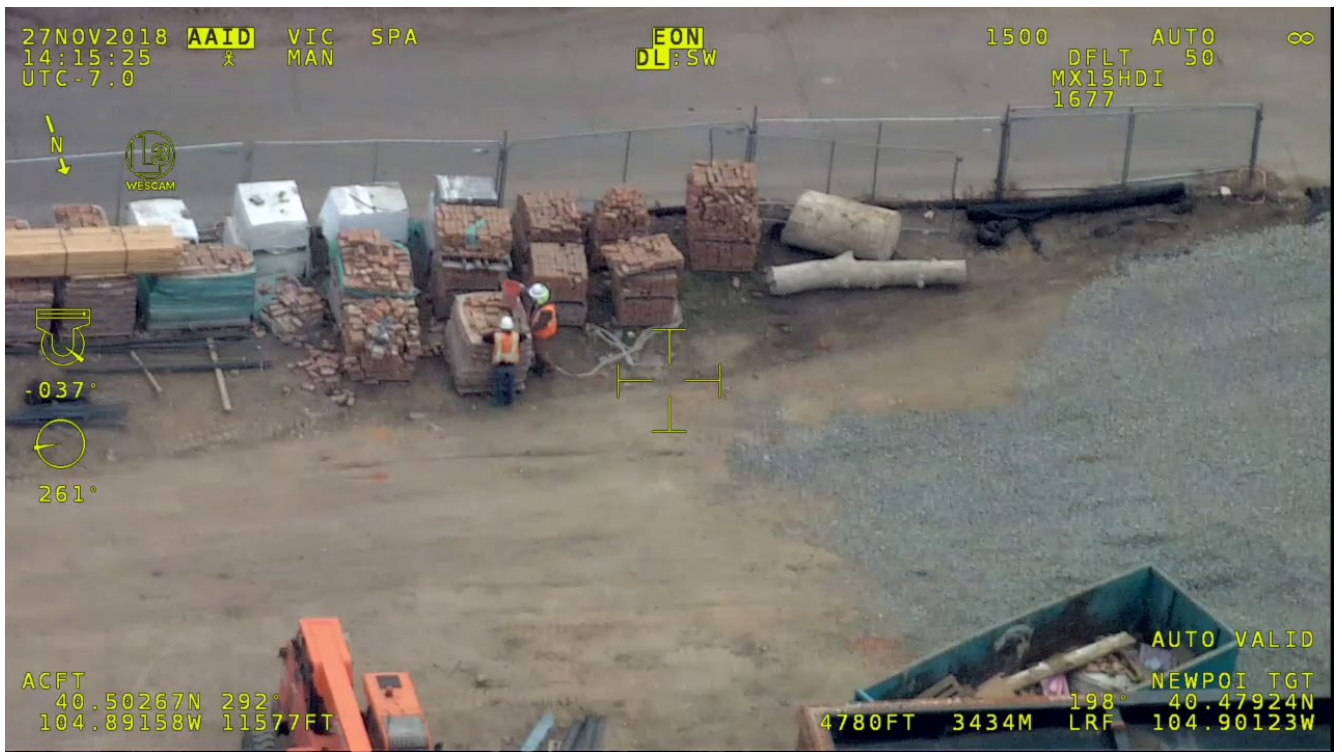
MX-15 from 6000 ft 3.4 km (1.8 nm) slant range EON
