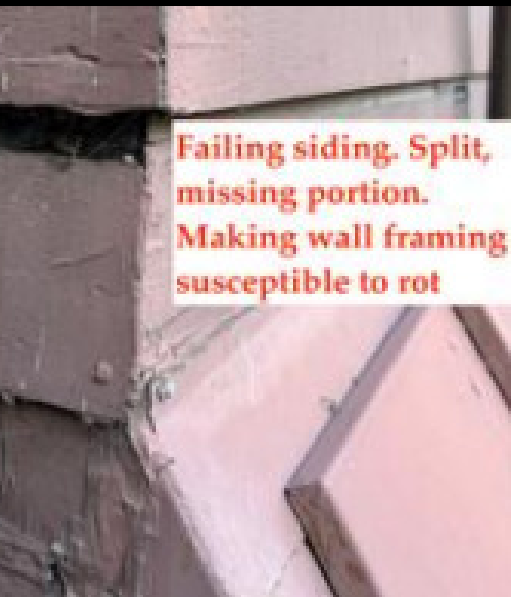
Example of failing shingles @ West face & ribbon coursing pattern
