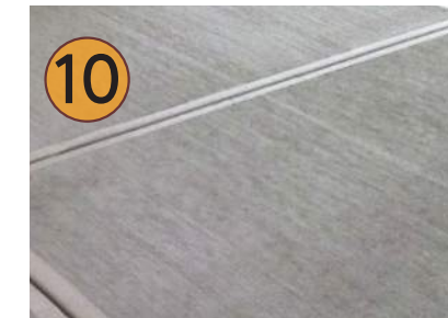
Existing Concrete Sidewalk
