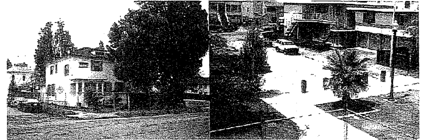
Fig. 4a Site Photographs: existing Community Center, 1999 (By PGA)
