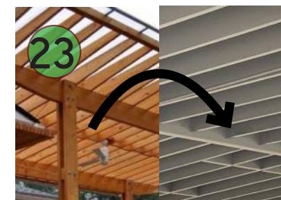
Wooden Pergola with Plexiglass (23) and "Enramada" (24); replaced by wood or metal frame and joist structure with polycarbonate parapet
