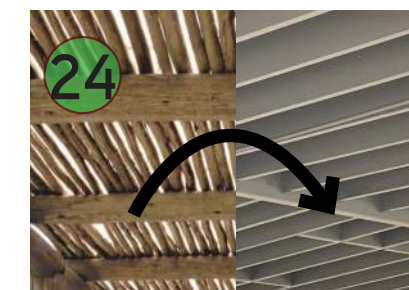
Wooden Pergola with Plexiglass (23) and "Enramada" (24); replaced by wood or metal frame and joist structure with polycarbonate parapet
