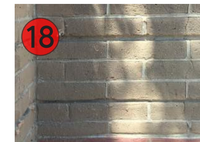
Adobe Brick Wall
