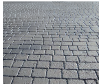
STAMPED ASPHALT PAVING
