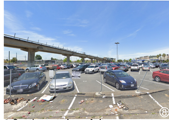
8-South west view of site
