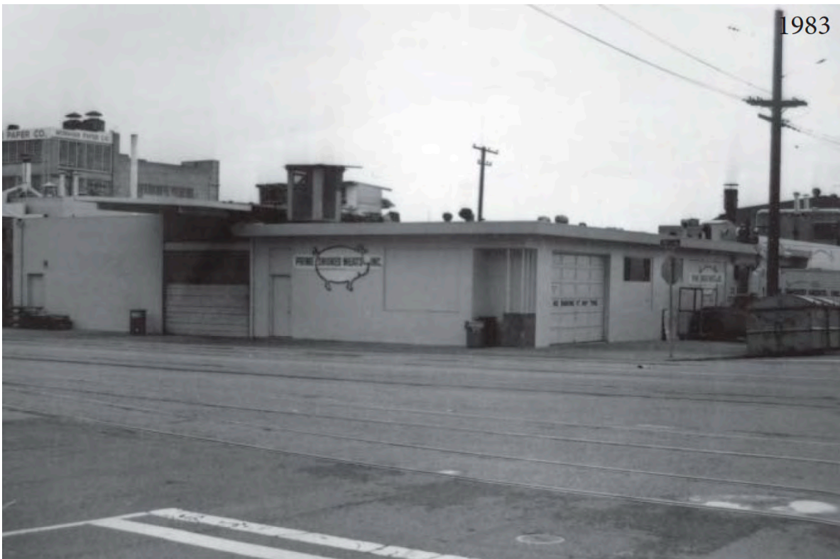
Figure 9: 220 Alice Street in 1983, corner café with pipe columns mentioned in the DPR forms is still visible (photograph courtesy of Carey& Co., Inc.)
