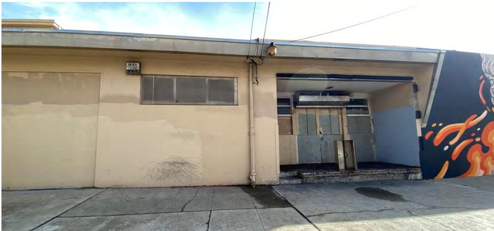
Figure 7: Alice Street Elevation, loading dock (Turnbull site visit December 2022)
