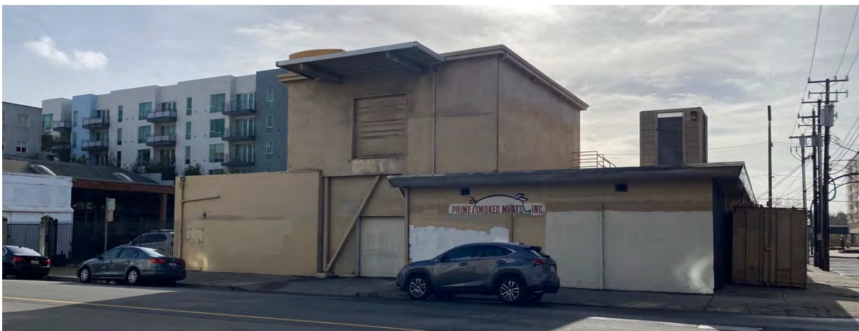
Figure 4: 3 rd Street Elevation (Turnbull site visit December 2022)
