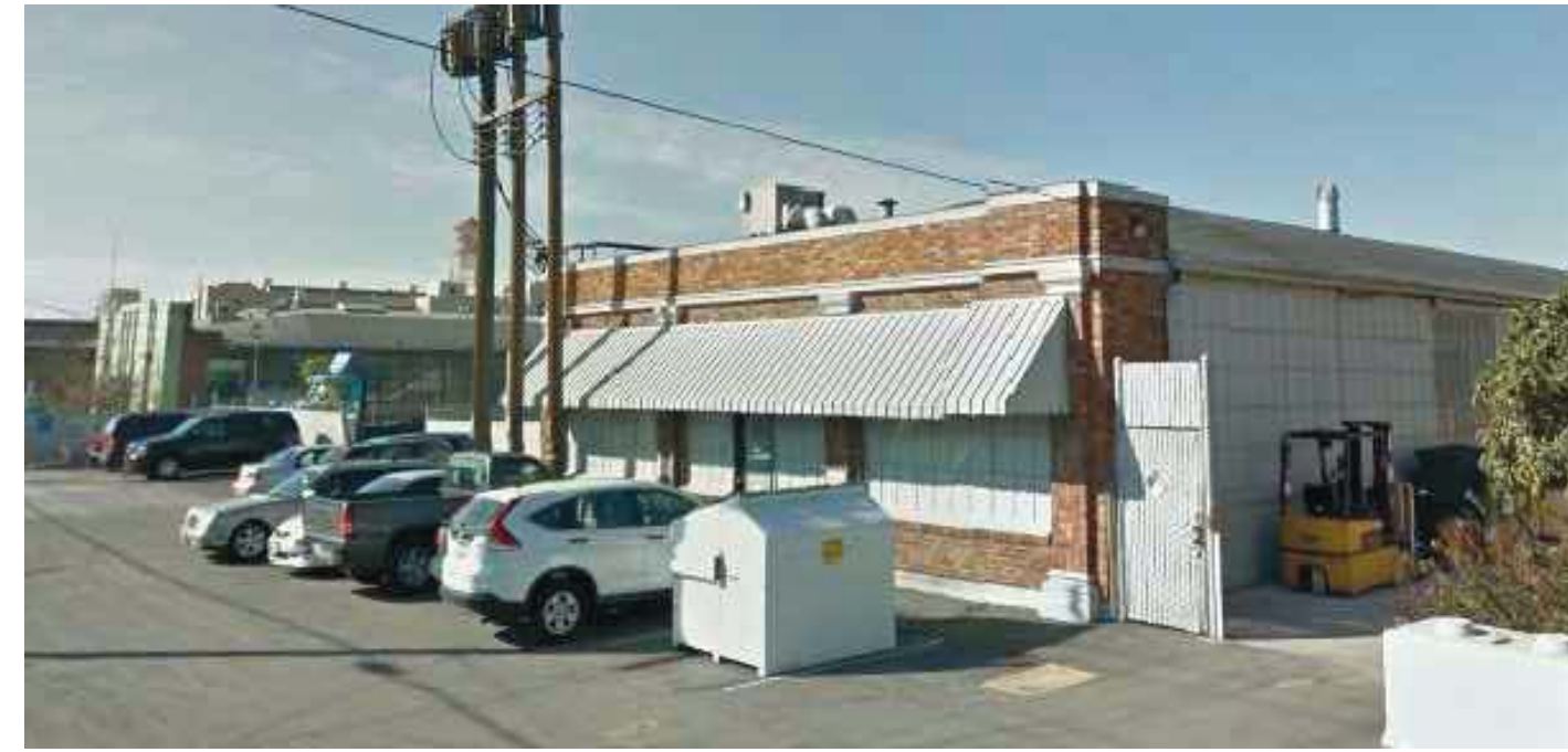
1127 57TH AVE. (NORTH)
