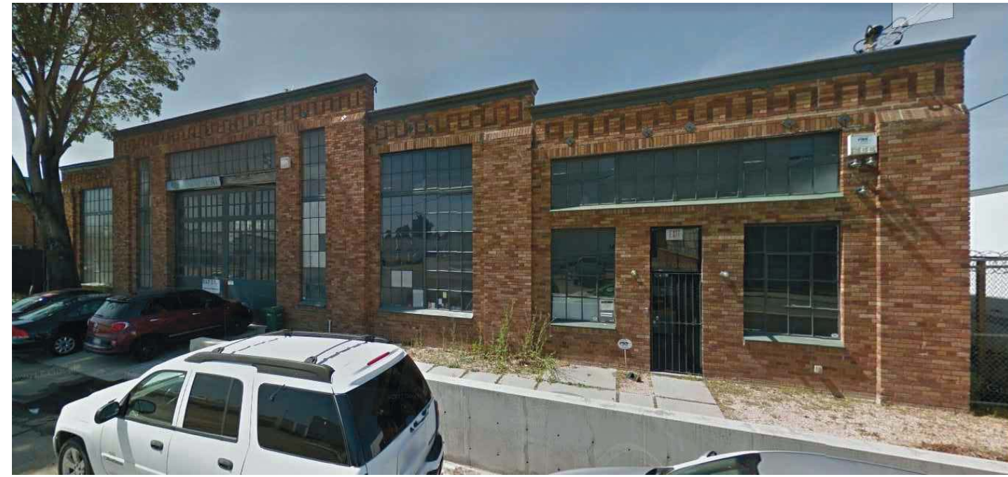
1137 57TH AVE., CONCRETEWORKS (NORTH)
