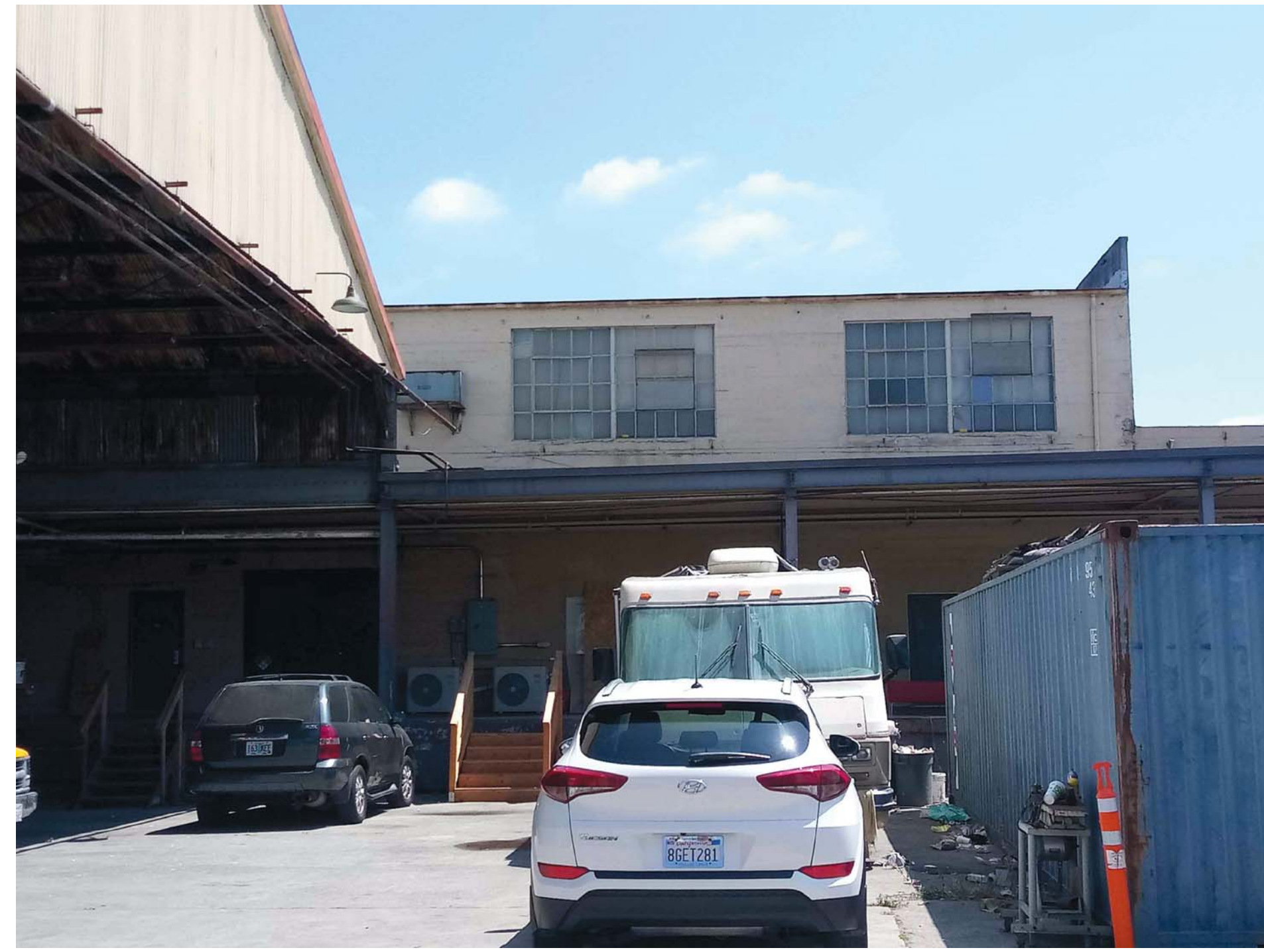
BUILDING K STEEL CANOPY OVERHANG
