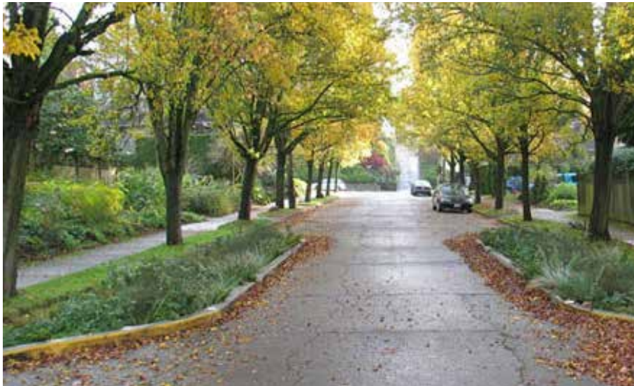
Integrated Stormwater Treatment - "Rain Gardens"
