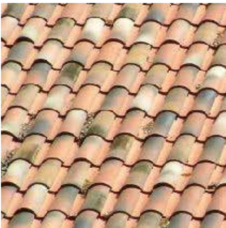
CLAY TILE ROOF
