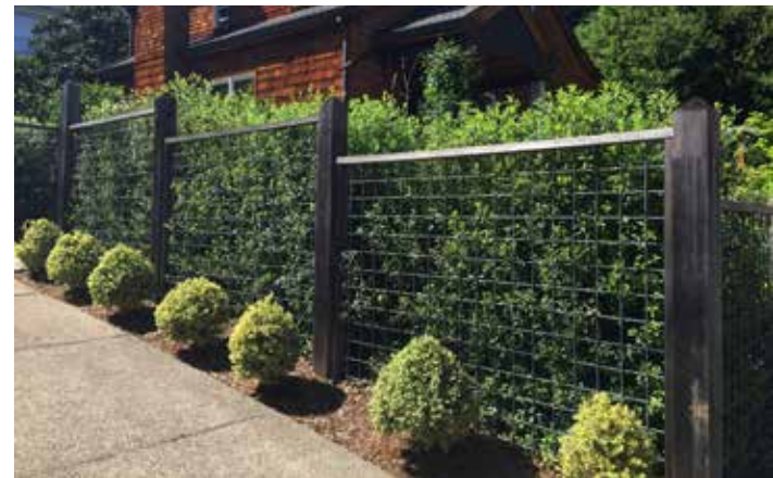
Typical Hillside Fence where slopes exceed 20% (stepped or sloping rear yard conditions)
