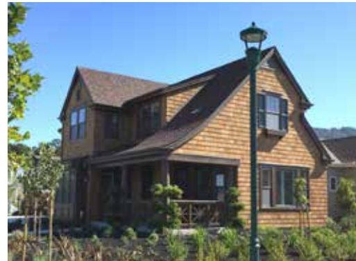
12/12 steeper pitch roof with dormers
