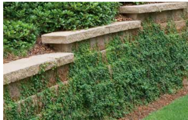
Vines planted on face of retaining wall
