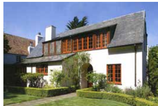
12/12 steeper pitch roof with dormers
