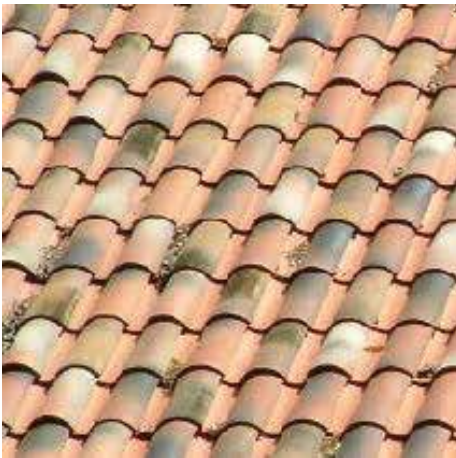
CLAY TILE ROOF
