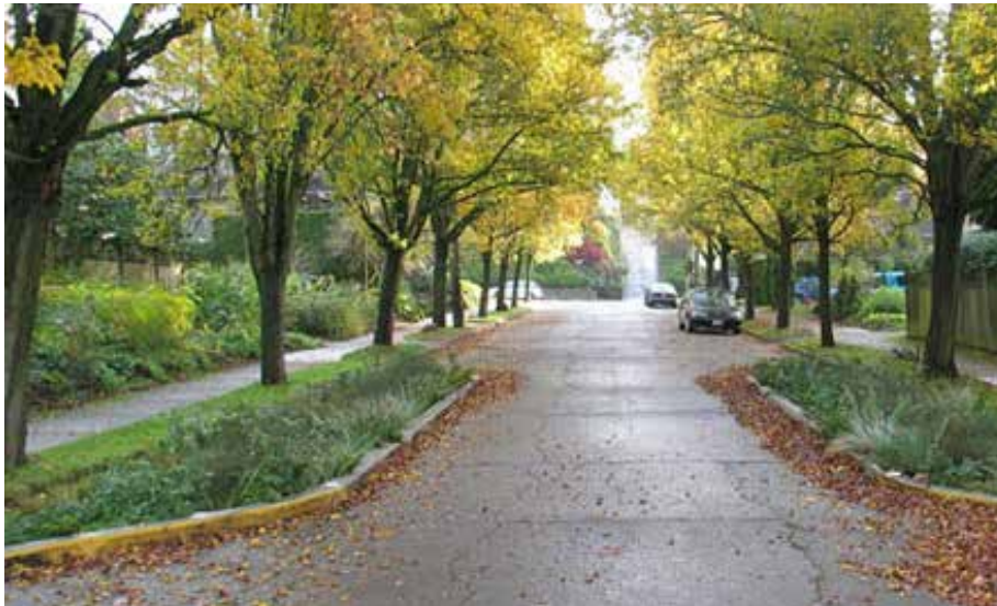
Integrated Stormwater Treatment - "Rain Gardens"
