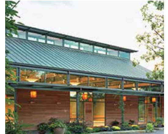
Clerestory Windows and Natural Lighting
