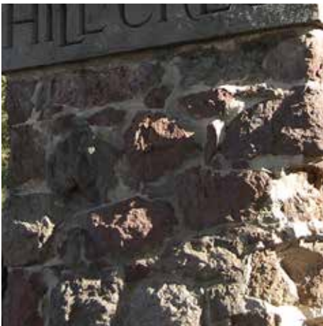
EXAMPLES OF ACCEPTABLE STONE VENEER FINISHES
