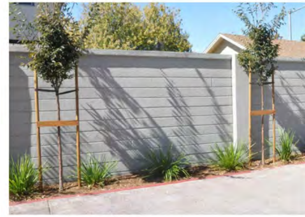
COMMUNITY WALL, CONCRETE PANEL, 6' TALL
