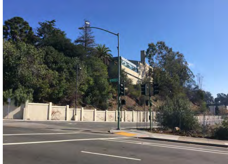
02 | View of Site and Access Road from Southwest
