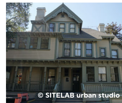
Figure 2.4: West porch (historical primary entrance) (above) and east porch to Macky Hall (below)
