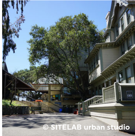
East of Macky Hall (view from northeast)
