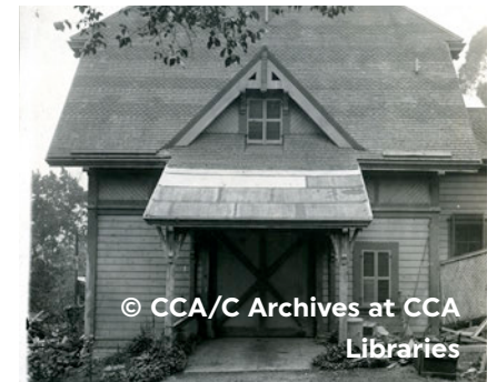
Figure 2.7: Carriage House original opening on east facade
