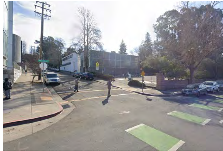
04 | Site View from Clifton & Broadway Corner
