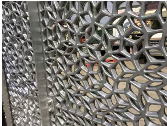
Cast aluminum as seen from the outside showing the fastening with mounting plates.
