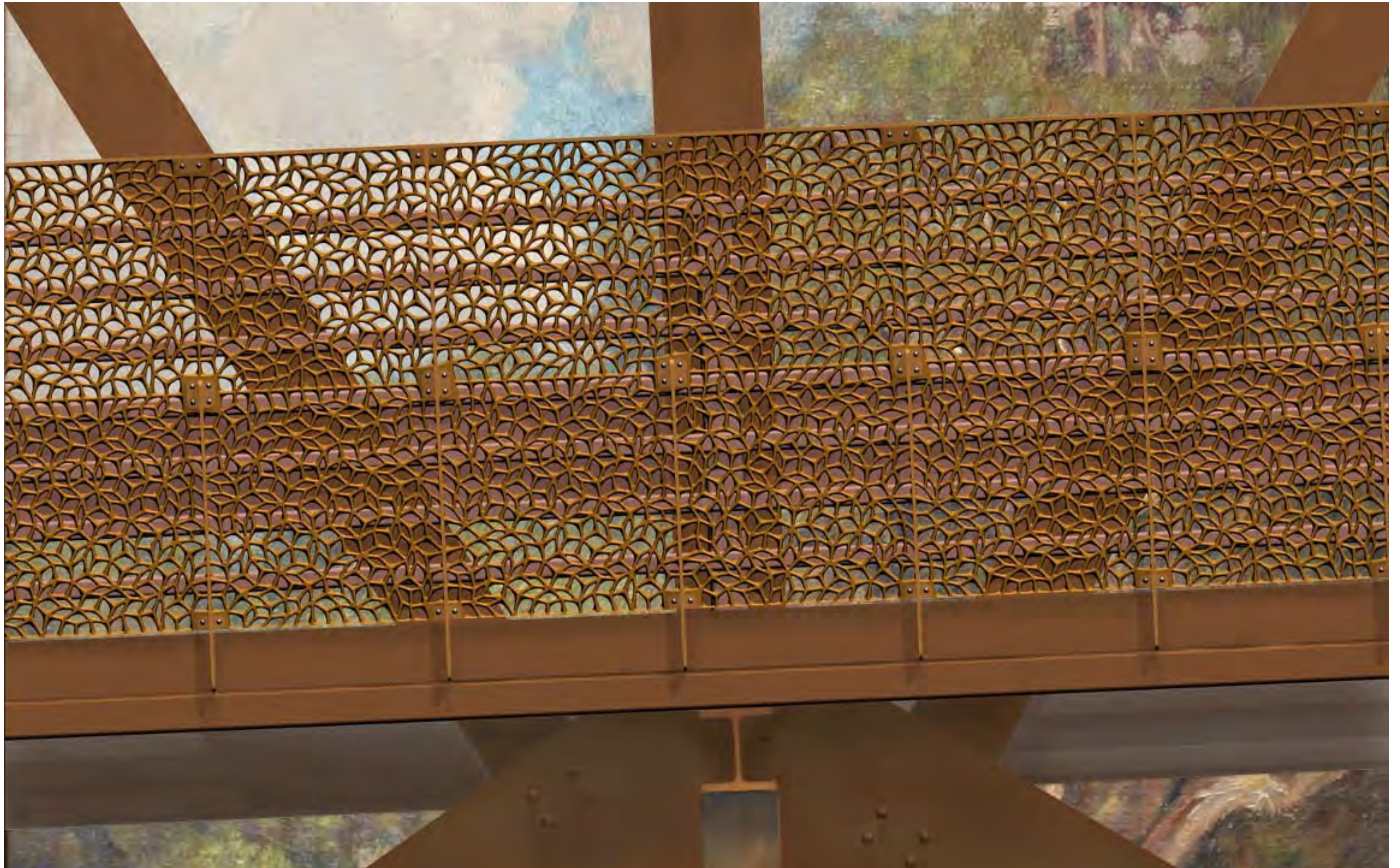
Oak Knoll Vehicle Bridge, North view detail, cast iron railing
