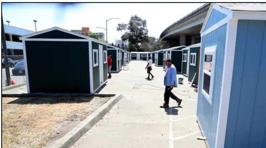
Figure 2. Community Cabin (Tuff Shed) Site.
