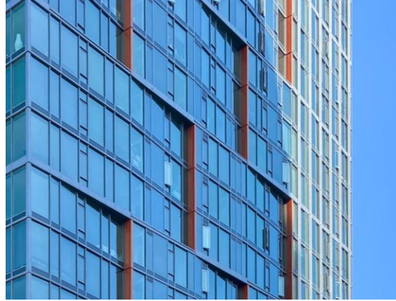
Modulation in Façade
