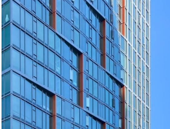
Modulation in Façade
