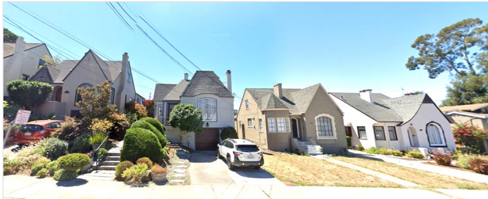
Neighborhood with strong roof context in Oakland Source: Google Street View
