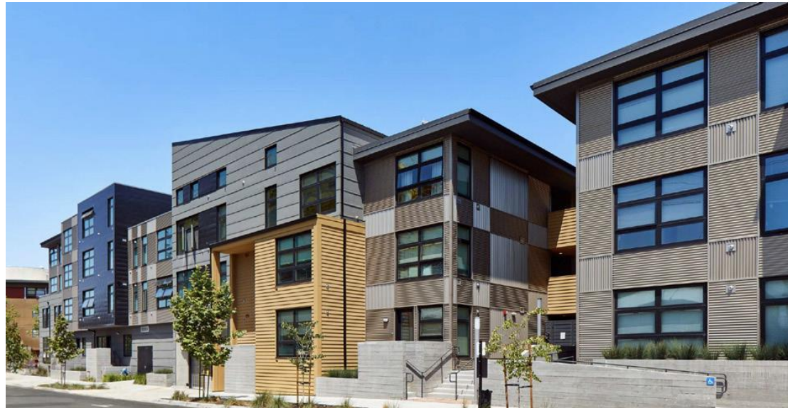
Recess and Projection in the building massing
