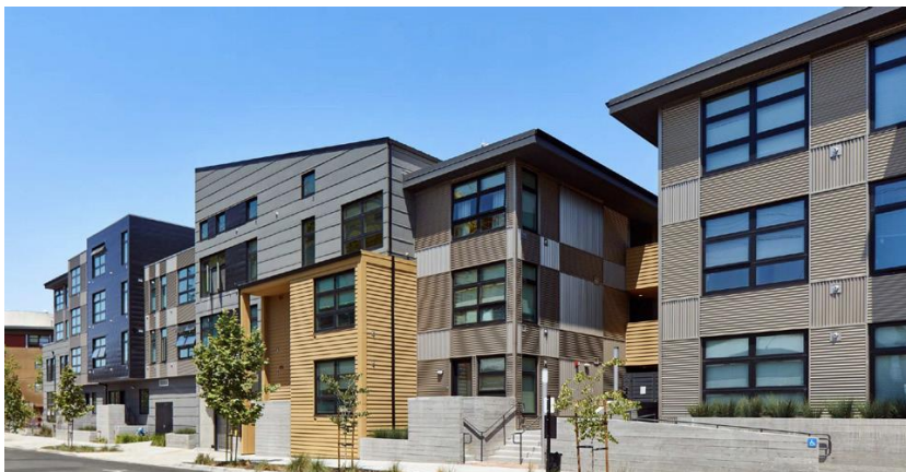
Recess and Projection in the building massing
