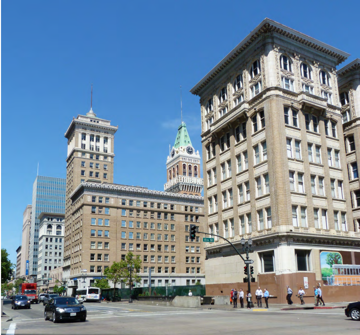
Oakland Downtown National Register Historic District: Before
