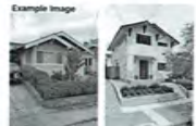
Example Image Front Articulation: Smaller roof forms, prominent ridge lines, and cornices or eaves at the roofline
