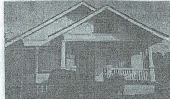
Fig. 8-8. The balanced use of multiple materials provide for houses well integrated into a context of either stucco or horizontally sided wood houses.
