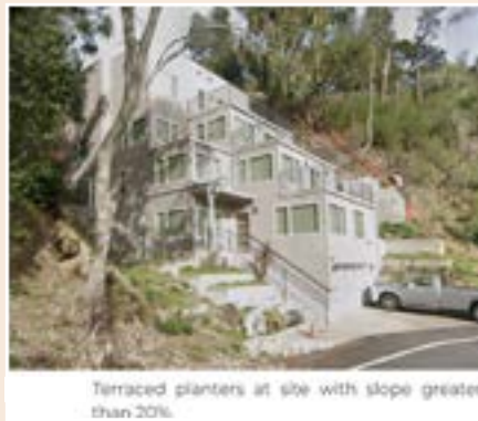
Planting provided to screen skirt walls at site with slope greater than 20%.
